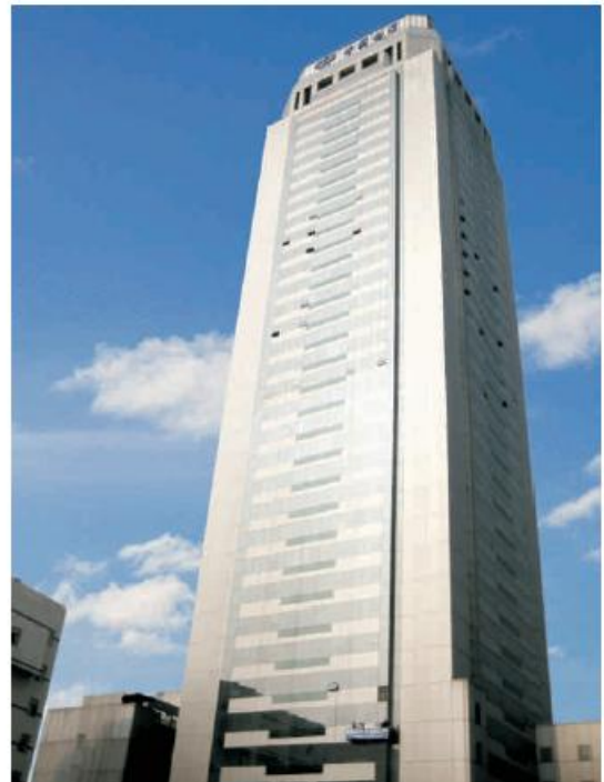
Jiangmen Branch Of China Telecom
